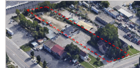
244 Mill Street, Kitchener
