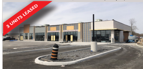
620 Dundas Street East, Belleville (Hwy 2)
