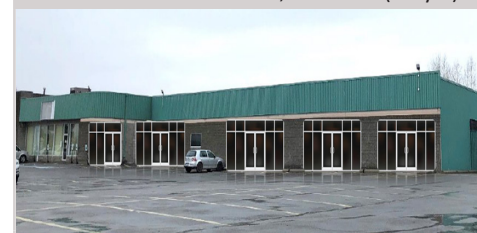
610 Dundas Street East #3, Belleville (Hwy 2)
